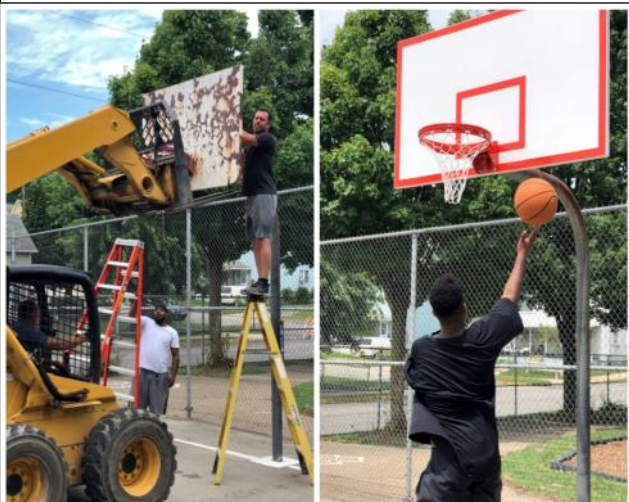
Before and After photos of restoration work on a playground!
